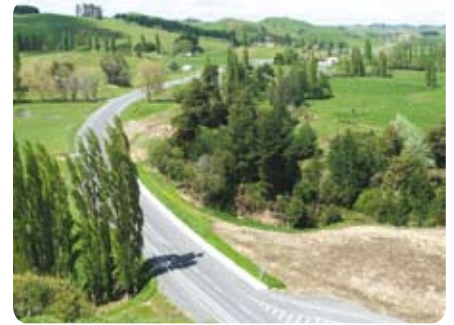
From the top of the northern bluff, looking south
