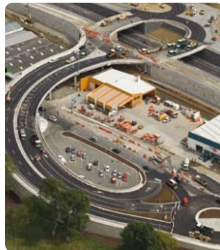
Dowse to Petone Interchange just before it was finished and opened
