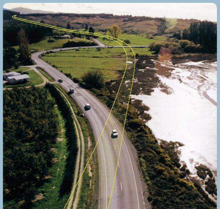
Dominion Road tie-in with the Ruby Bay Bypass.
