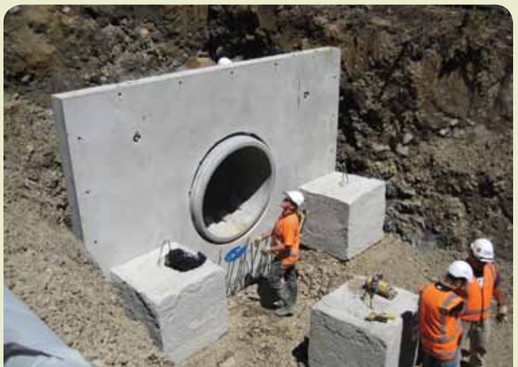
The energy dissipation unit is assembled on site using pre-cast sections.
